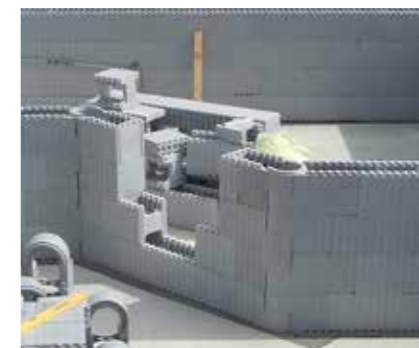
The use of hinge elements to shape corners at any angle.
