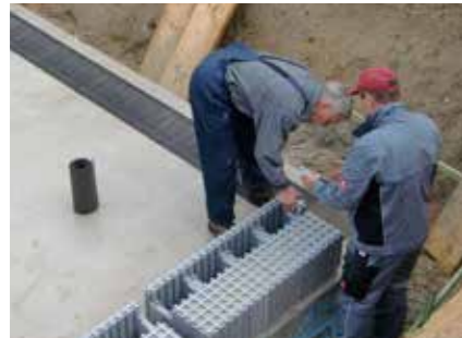
The first layer of elements.
