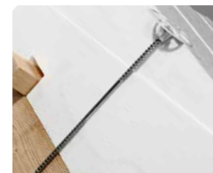
Expansion bolt used to fix the Izodom roof slab.
