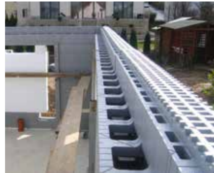
The MP ring beam element has an external insulation layer, which is the same as in the entire wall.
