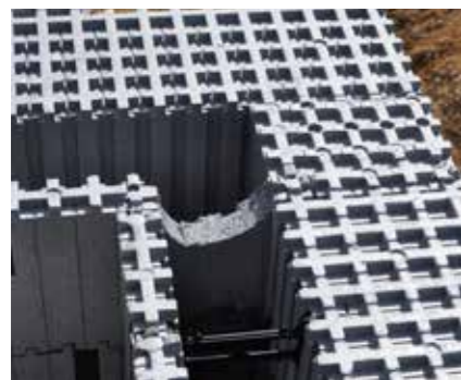
When a portion of the element is removed, continuity of concrete filling will be obtained.
