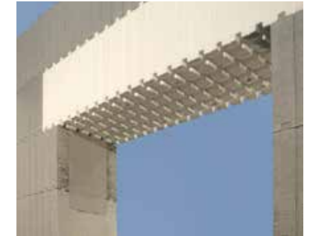
The header element has a U-shaped cross-section.
