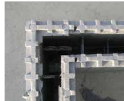
MCF 1/15 element at the corner.
