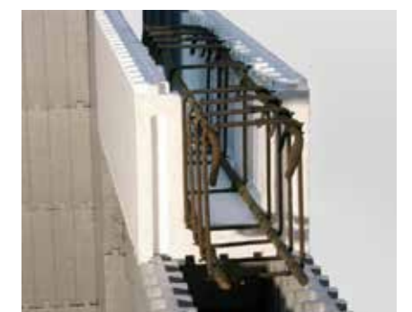
Placement of reinforcement in the ML header element is simple.
