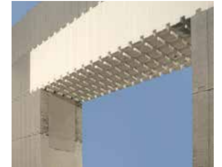
The header element has a U-shaped cross-section.
